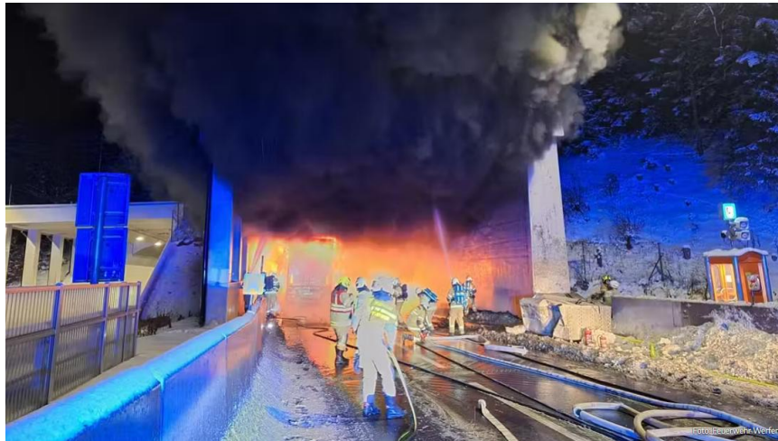
Brand Brentenbergtunnel Tauernautobahn 09.01.2026
